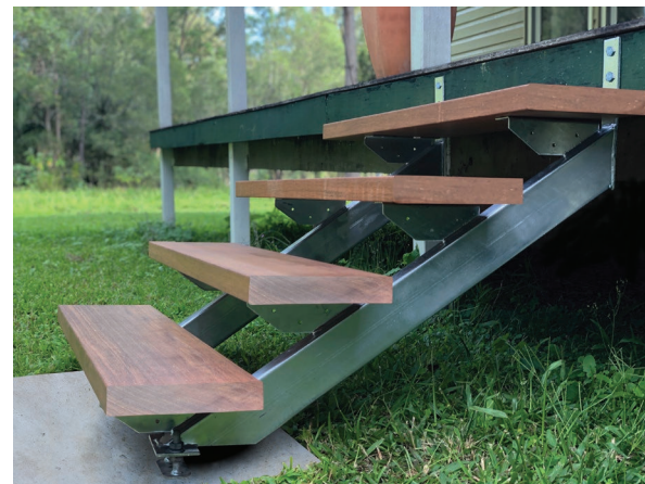
4T-SSBD installed with Merbau Treads.
